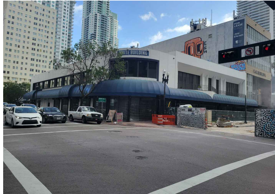
Existing Site Photograph
