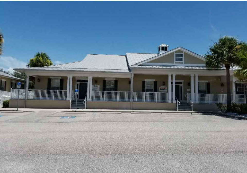
Existing Site Photograph
